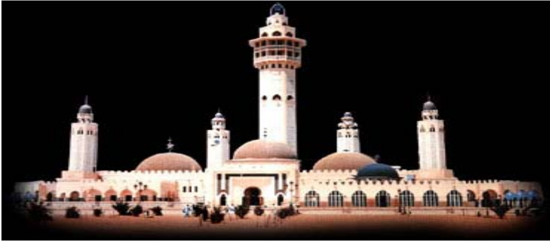
The Touba Mosque: one of the largest on the African continent
